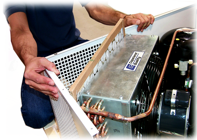
Figure 84: Replacing the Air Filter
