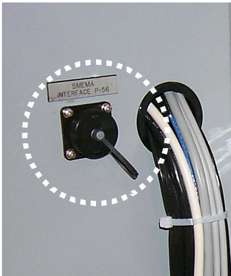
Figure 14: SMEMA Connector (Load End)
