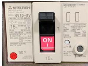
2. Change the **Main Switch** on the left side of the machine to **ON**.
