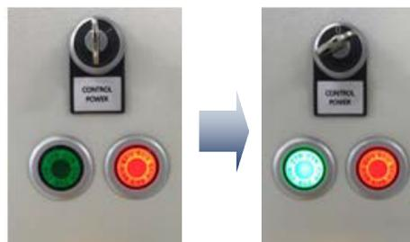
6. Check that the **Control Power Lamp** is **ON**.
